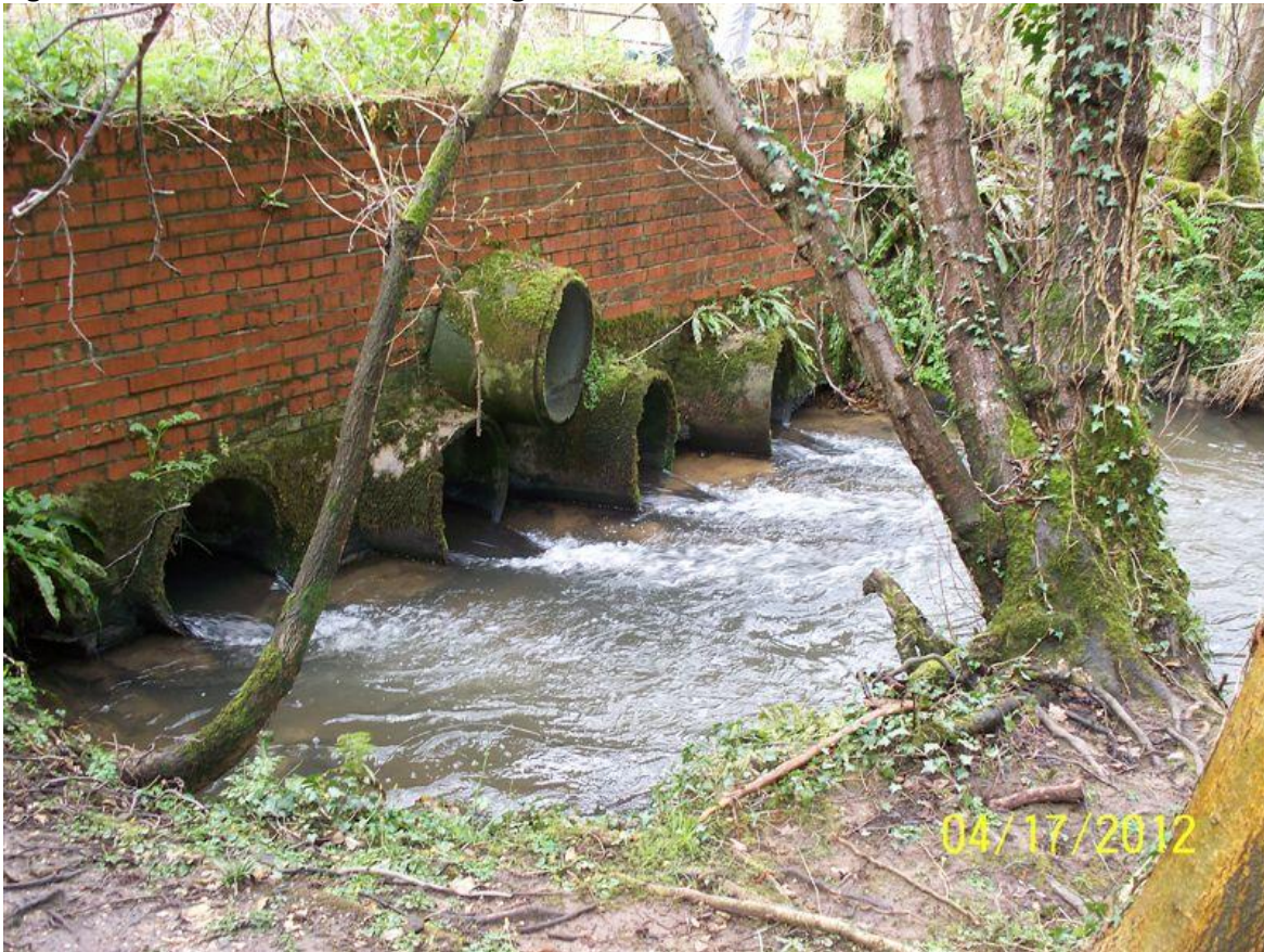
Figure 7: the multi-culverted farm bridge over the Costers Brook SU 89432 20135
